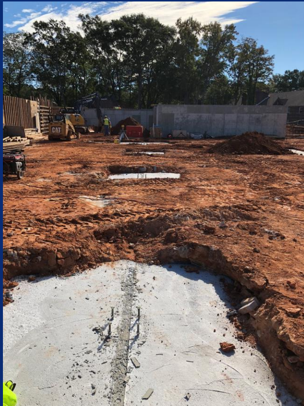
Spread footings poured for temporary steel
