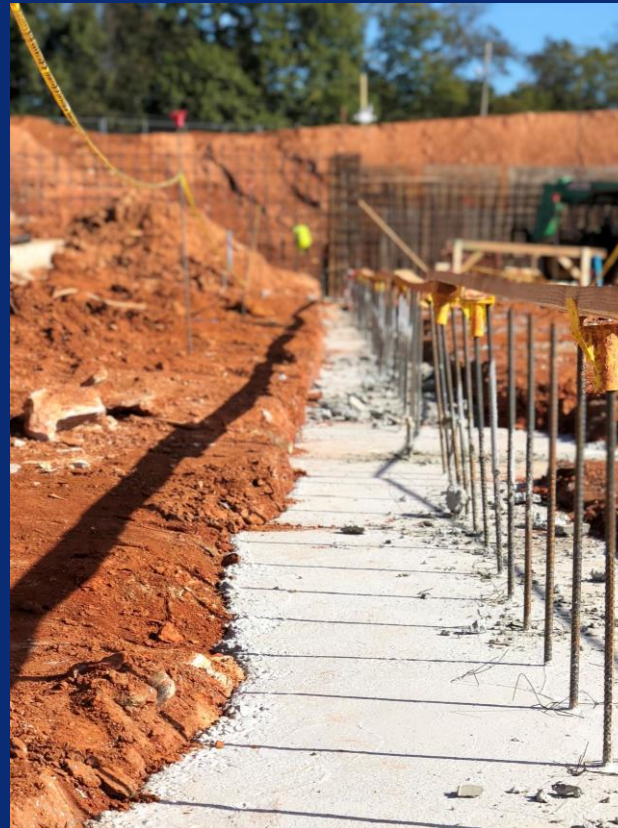
Footings poured for CMU wall at gymnasium and kitchen
