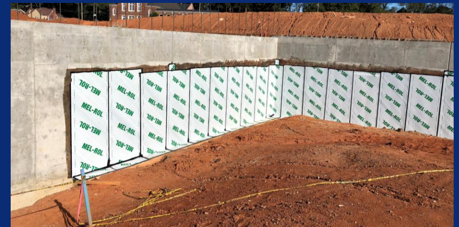
Below grade waterproofing at southeast corner of building
