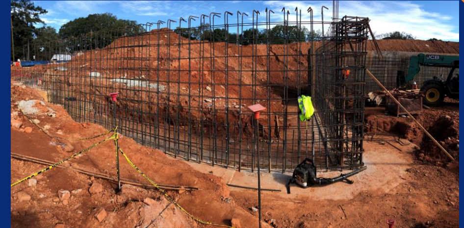
Retaining wall reinforcement and forming west of gymnasium
